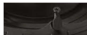
Stainless steel fixing screws with Neoprene covers
